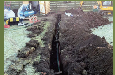
INSTALLATION OF WATER TREATMENT EQUIPMENT
