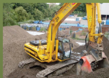
TURNING OF CONTAMINATED SOILS
