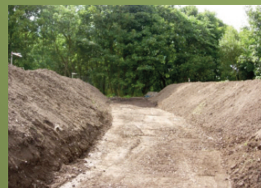
INITIAL EXCAVATION AND DUMPING OF STOCKPILED SOILS
