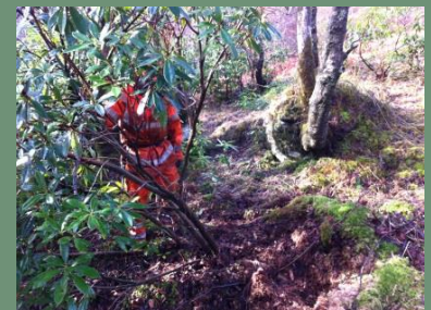
MANUAL REMOVAL IN OPERATION
