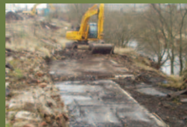
SCRAPING BACK SOILS ALONG THE CANAL BANK
