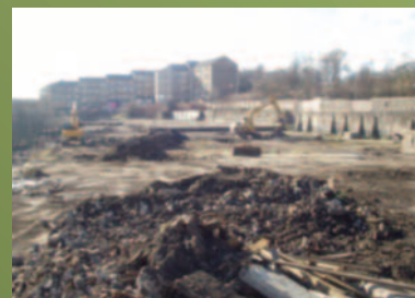
SOIL AND DEMOLITION MATERIAL ON SITE
