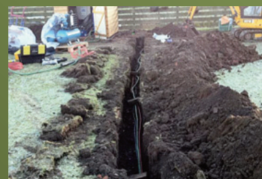
INSTALLATION OF WATER TREATMENT EQUIPMENT
