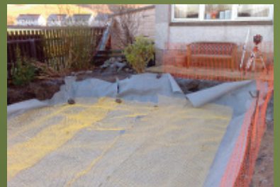
INSTALLATION OF TEXTILE AND 'GEO-GRID' PROTECTION PRIOR TO BACKFILLING.
