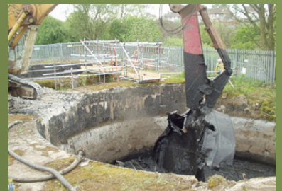
EXTRACTION OF SCRAP FOUND IN 1 TANK
