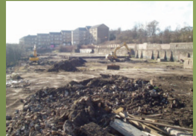
SOIL AND DEMOLITION MATERIAL ON SITE
