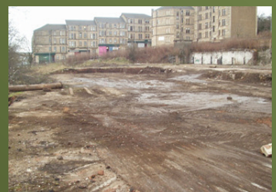
CLEARED AREA OF SITE UPON COMPLETION OF WORKS
