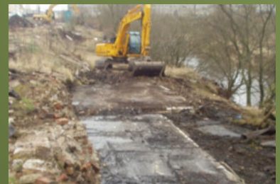
SCRAPING BACK SOILS ALONG THE CANAL BANK
