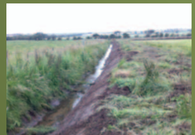
DRAINAGE TRENCH FOLLOWING EXCAVATION WORKS
