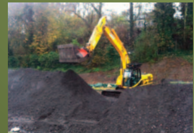
'TURNING' OF WINDROWS USING AN ALLU BUCKET
