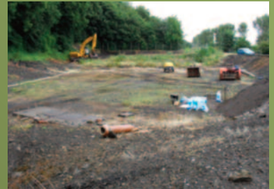
REMEDIATION AREA AT THE START OF WORKS
