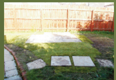
FINAL RE-INSTATEMENT PRIOR TO TANK INSTALLATION.
