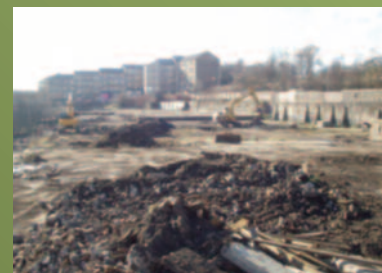
SOIL AND DEMOLITION MATERIAL ON SITE
