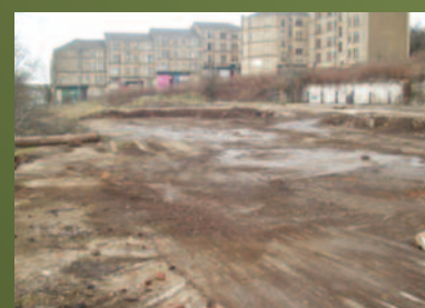
CLEARED AREA OF SITE UPON COMPLETION OF WORKS
