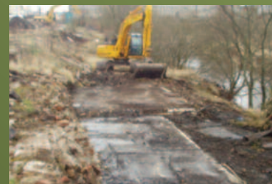
SCRAPING BACK SOILS ALONG THE CANAL BANK
