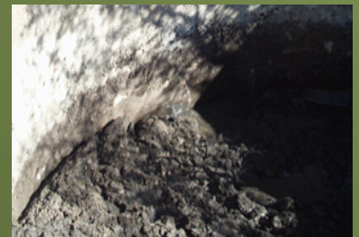
MATERIAL FOLLOWING STABILISATION
