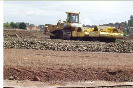
Engineered capping layer prior to development of a residential housing estate.
